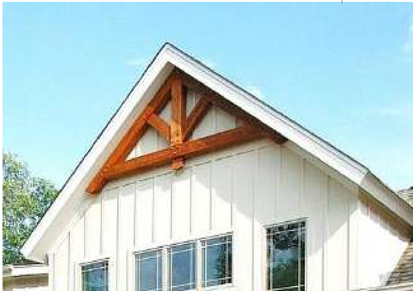
TRUSS IN GABLE
