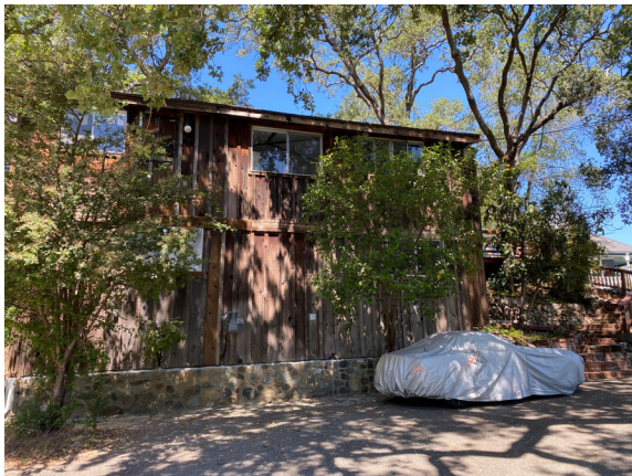
Existing two-story ADU to be demolished
