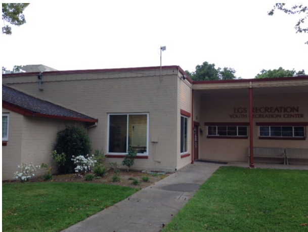
C Youth Recreation Center Roof Repair
