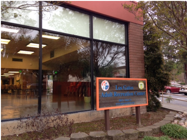
D Adult Recreation Center Cable & Control System Repairs
