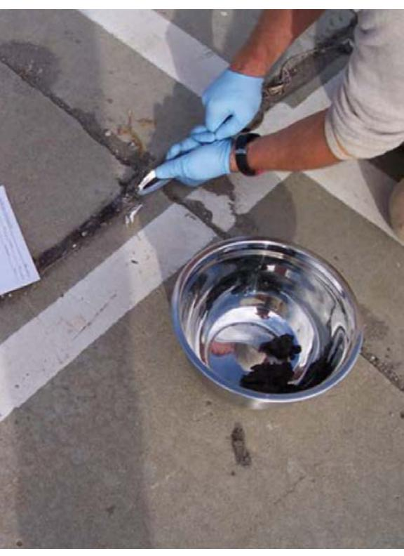
A photograph showing a person's hands wearing blue gloves. They are using a tool to apply a dark, viscous material, likely caulk, into a concrete expansion joint. A metal bowl is placed on the floor next to the joint, reflecting the surroundings. The floor is made of concrete with white diagonal stripes. |
