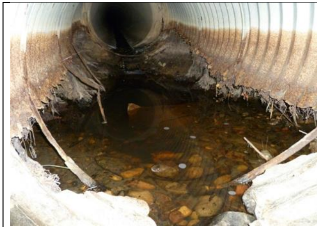
D Bicknell Road Storm Drain Improvements
