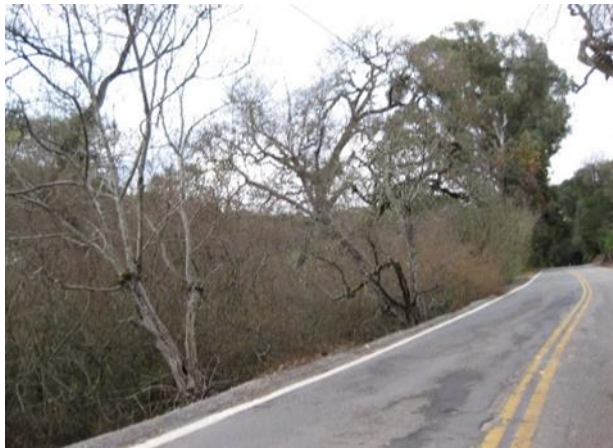
B Guardrail Replacement
