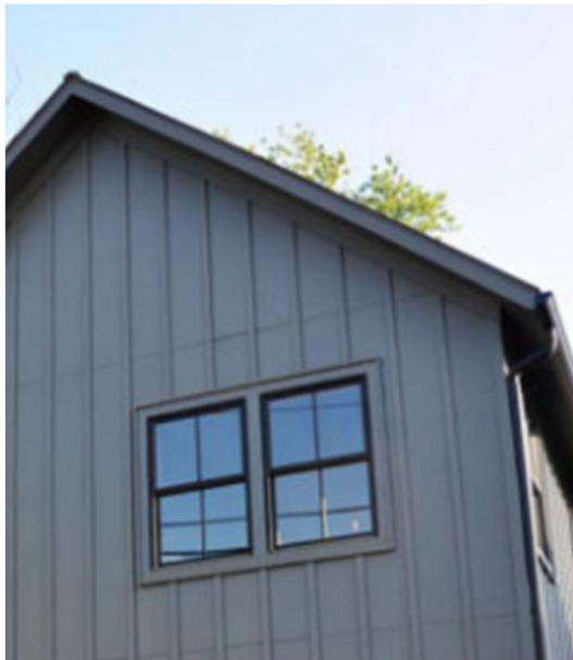
WINDOW, KOLBE ALUMINUM GLAD, ULTRA SERIES, COAL BLACK
