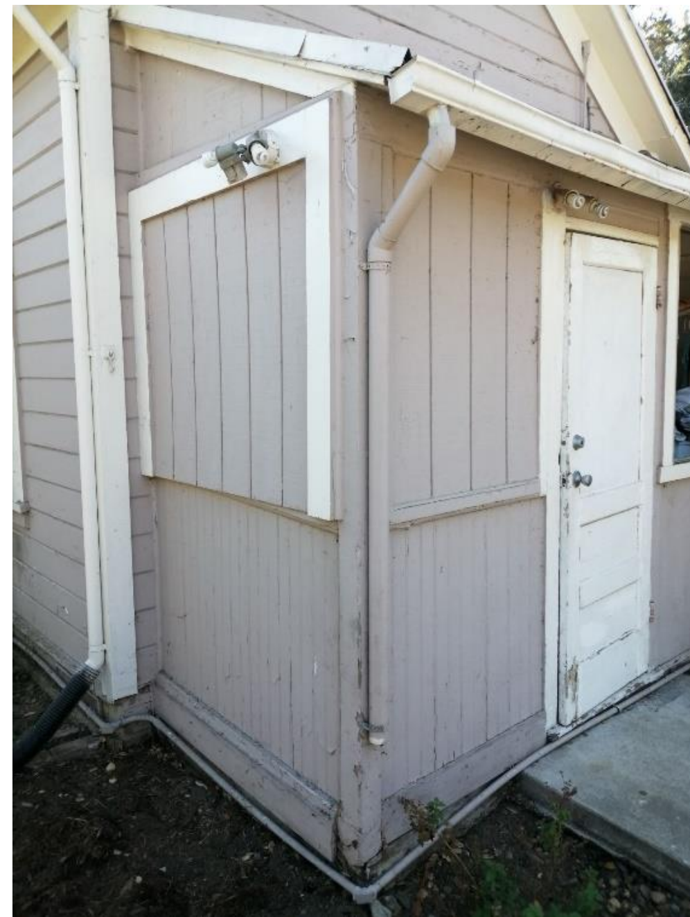
REAR NORTH-WEST CORNER
