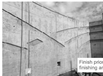
Patterns and lettering formed by field-cut plywood shapes and chamfer strips attached directly to forms (Santa Clara Caltrain Station). Since shapes are field cut from plywood, any shape can be used. Edges are beveled to improve finish at corners
