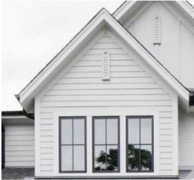
Painted corner board trim + painted trim @ wall to roof connections, profile TBD. Horizontal wood siding.
