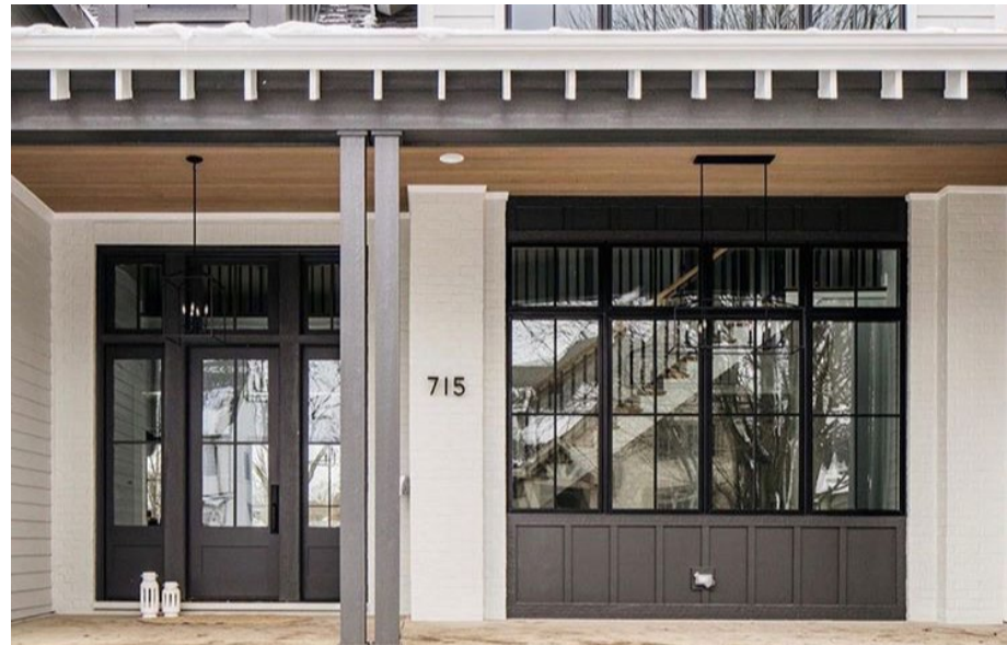
Stained wood posts + beam. Exposed rafter tails.
