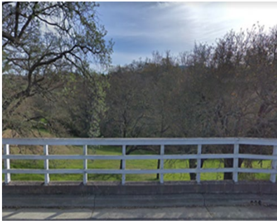
B Fence Replacement – Shire Court
