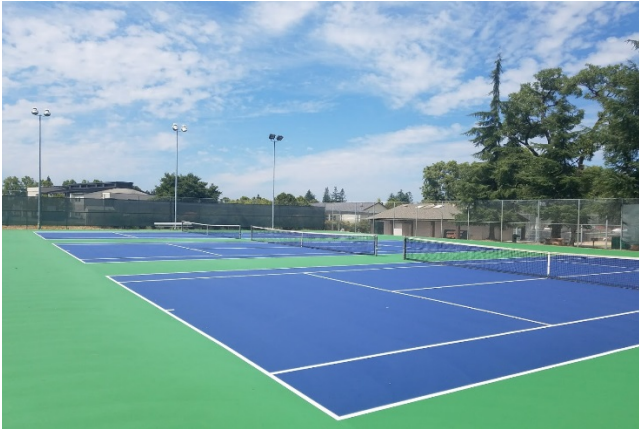
D Tennis Courts Repairs – Various Town Parks
