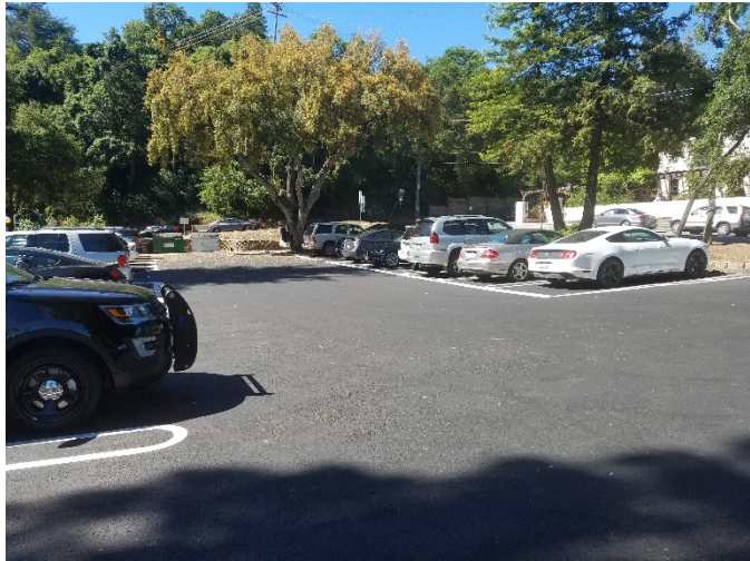
A Pageant Way Parking Lot Reconstruction
