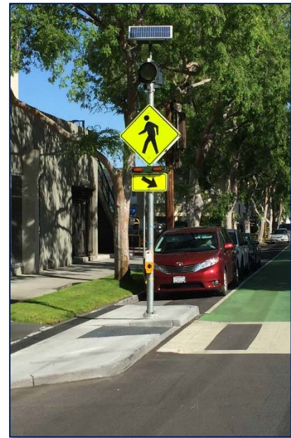
3-Section Pedestrian-Activated Flashing Beacon Solar Powered
