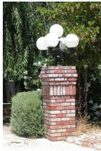
Inappropriate lighting fixture
