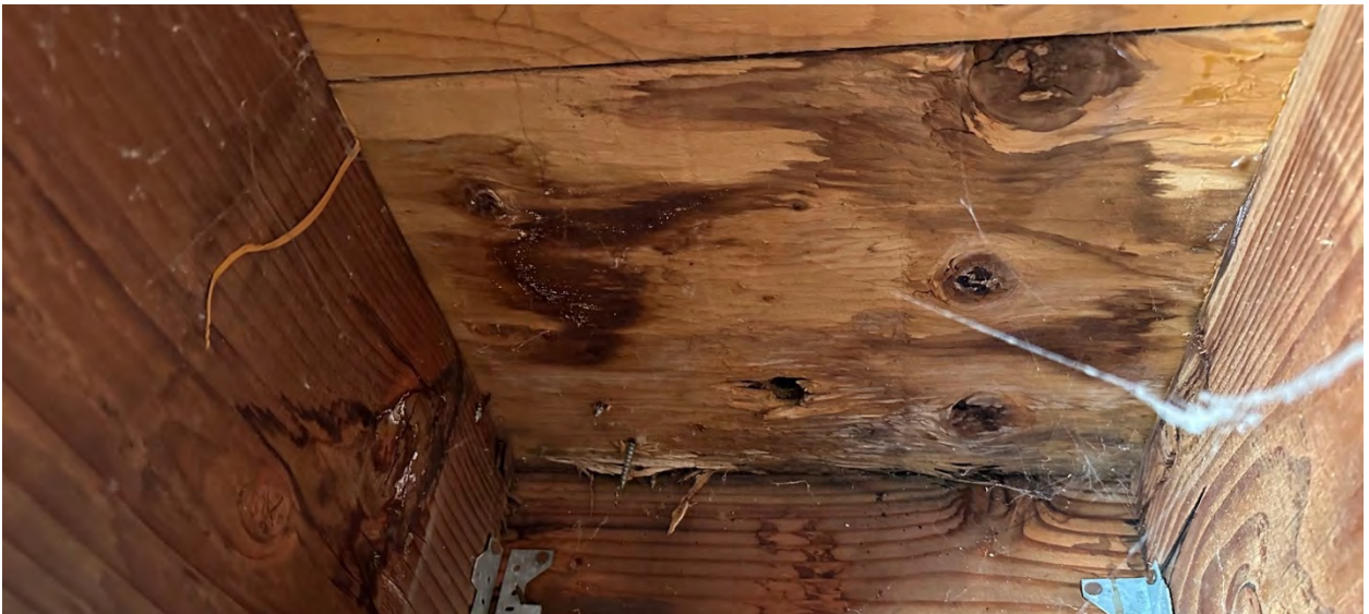
Water damage and rot in substructure as seen from inside the garage below
