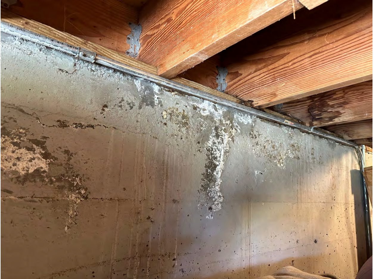
Water is entering concrete wall below
