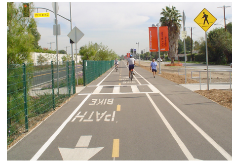
Example of a multi-use path with separate pedestrian zone
