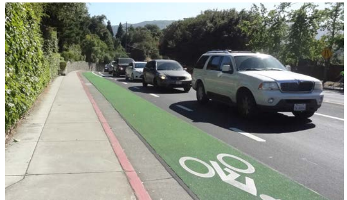
Green Painted Bike Lane on Blossom Hill Road at Roberts Road East.
