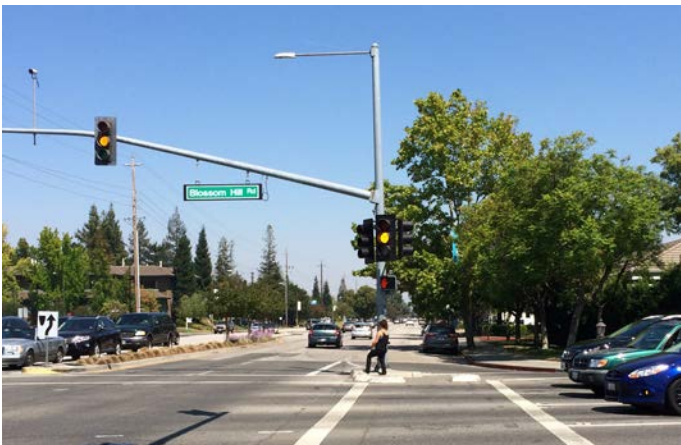
Pork chop intersection at Blossom Hill Road and Los Gatos Boulevard (looking north from Los Gatos Boulevard).
