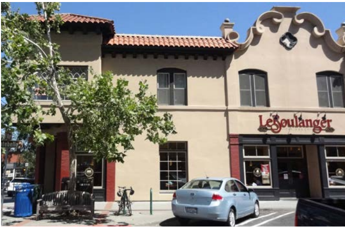
Downtown Los Gatos consists of a mix of land uses with 1-3 story buildings.
