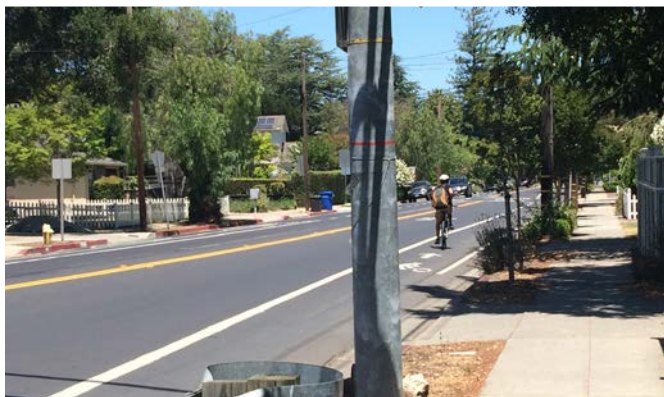
Bike lane on Los Gatos Boulevard with striping on both sides.
