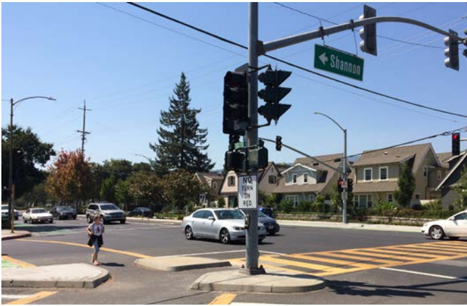
Pork chop intersection at Shannon Road and Los Gatos Boulevard (looking south toward Los Gatos Boulevard). This intersection is heavily used by bicyclists and pedestrians, with many crossing Los Gatos Boulevard at Shannon Road to get to Van Meter Elementary School and Fisher Middle School.
