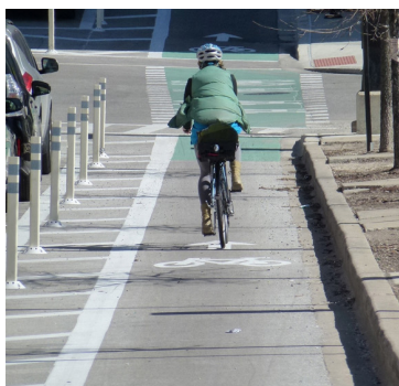
Cycle track with posts and painted buffer
