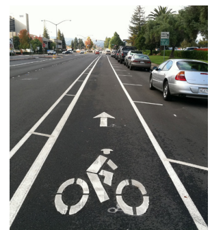
Example of a two-sided buffered bike lane demarcating a path outside the parked vehicle "door zone"
