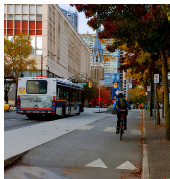
Raised pedestrian crossing at cycle track
