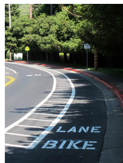
Example of a curbside buffered bike lane providing separation from the vehicle travel lane
